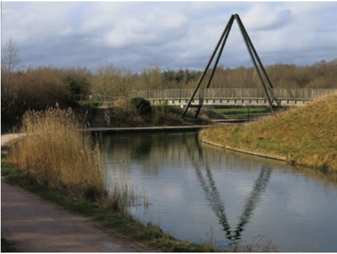
Ashby Canal & Marquis Bridge
